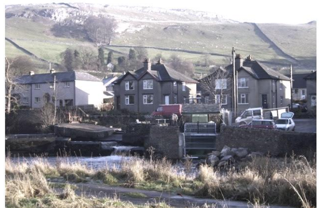
The hydro system in place in Settle
