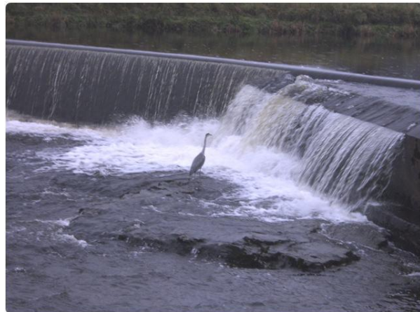
The Hydro generator works in harmony with local wildlife
